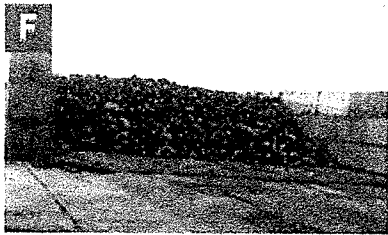
▲ Straight front (blunt) bunker walls. Note that wooden 2x4s are used as a 'stop' to prevent rolling bottles; these boards are easily removed for loading.
